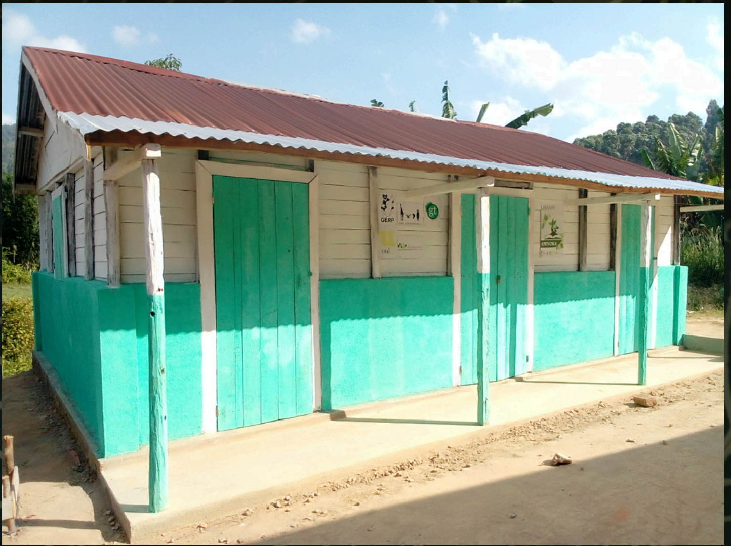
Santi's House after the renovation
